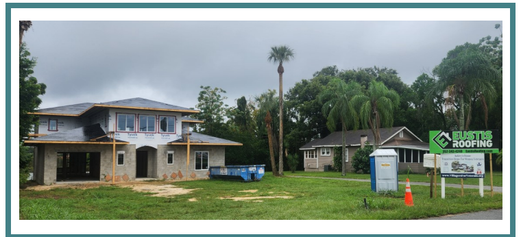
Eustis Roofing is under contract to complete the roof.
